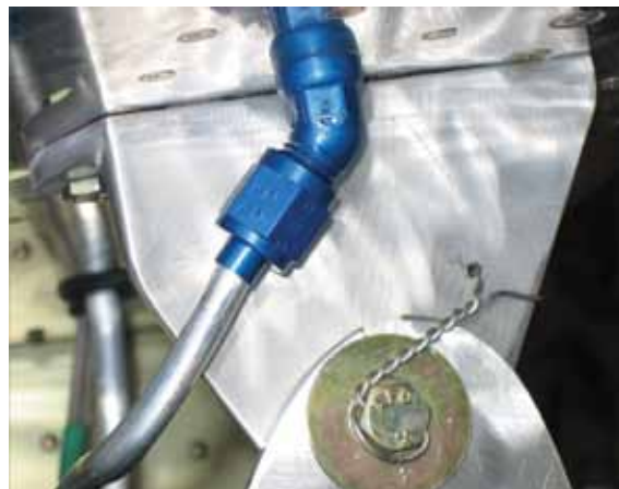
It’s a pretty fuel-line installation, but it wasn’t quite right. The tube had to be remade because it was rubbing on the large bracket. All it took was a slight kink to make it better.
